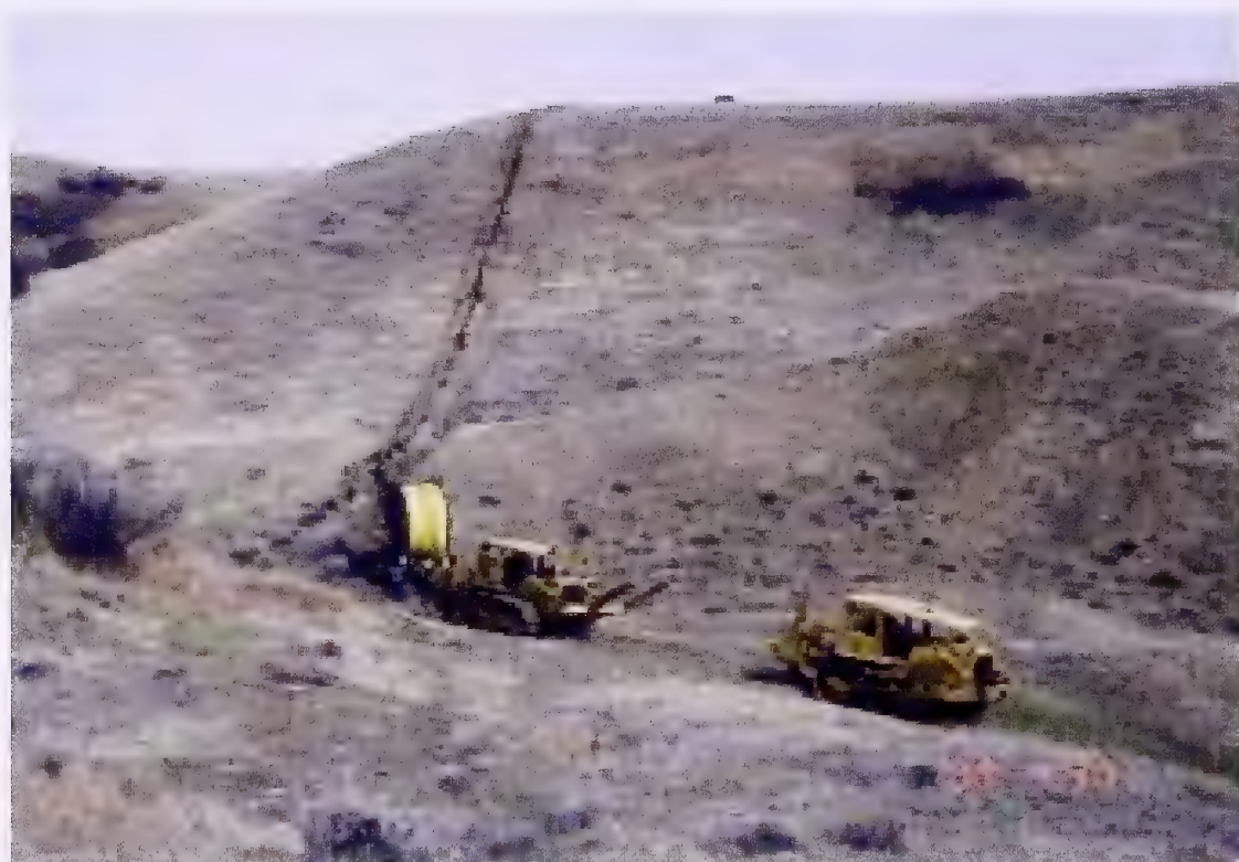
Photo 18 Minimizing disturbance with small diameter pipe
